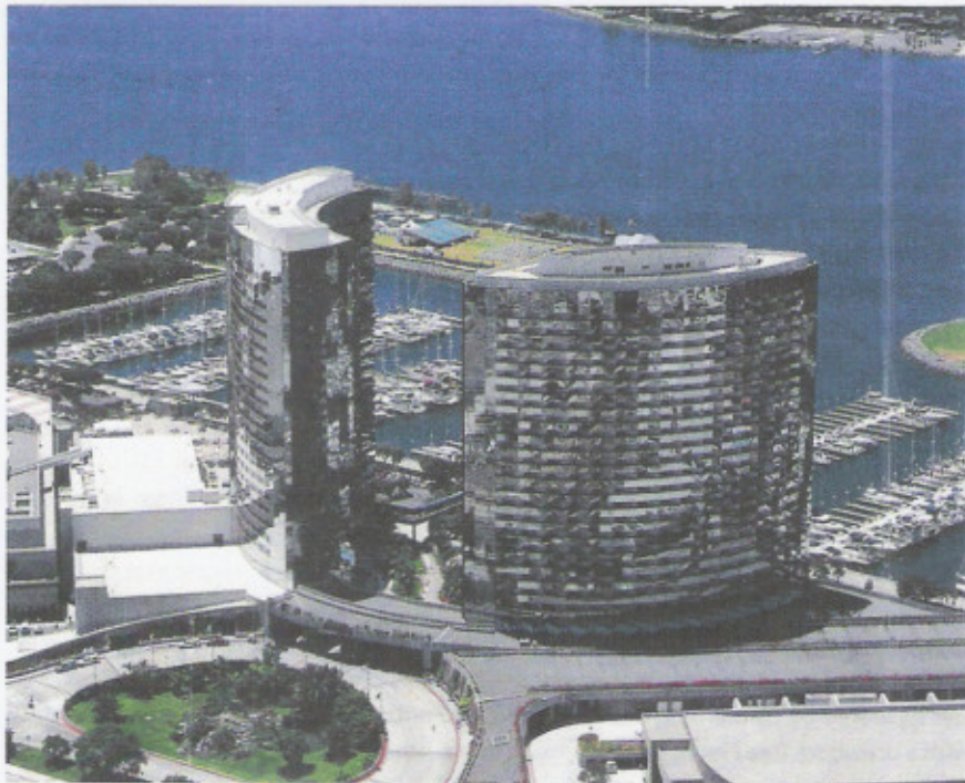
Figure 1. The San Diego Marriott Hotel and Marina, home of the boiler replacement project discussed in this article. The South Tower is the high rise on the right side of the picture. Photo: San Diego Marriott Hotel and Marina
